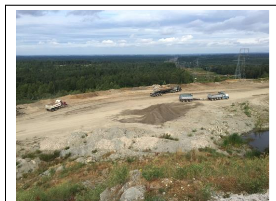
Backfilling operations at the Ravensdale site. (reservesilica.com)
